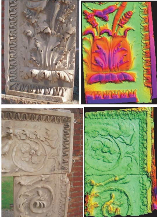
Figure 5: Detailed ornaments modeled by means of dense image matching and derived surface models shown in colour-code mode.
